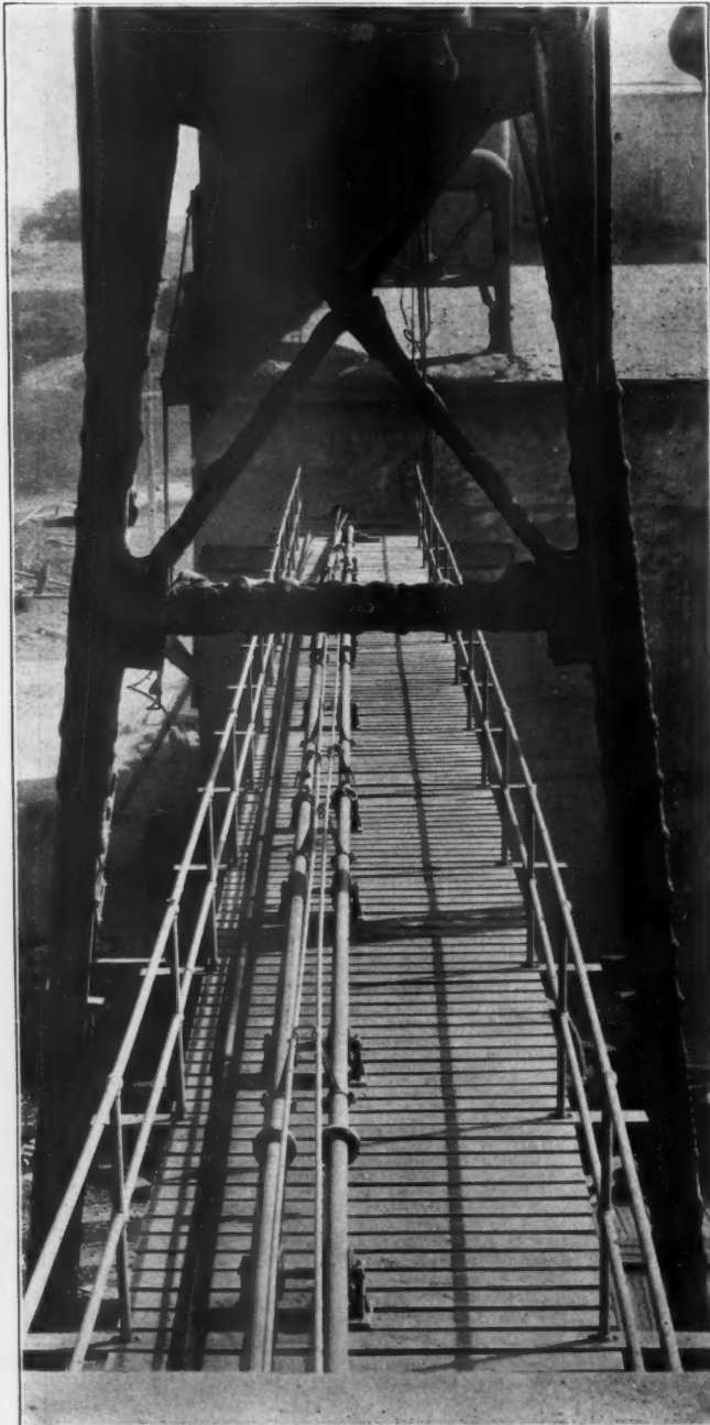
Pipe Line Conveying Cement to Stock House
